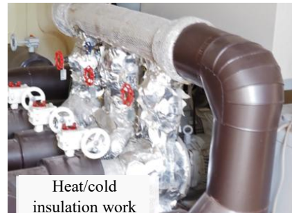
Heat/cold insulation work
