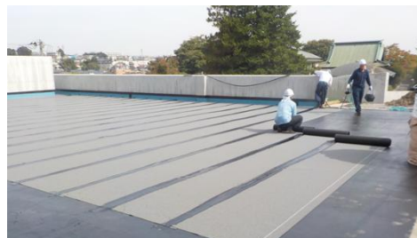
Yopishtirish usuli (asfalt tol ruloni yordamida gidroizolyatsiyalash)
