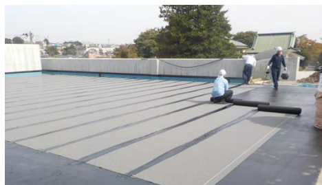
Yopishtirish usuli (asfalt tol ruloni yordamida gidroizolyatsiyalash)
